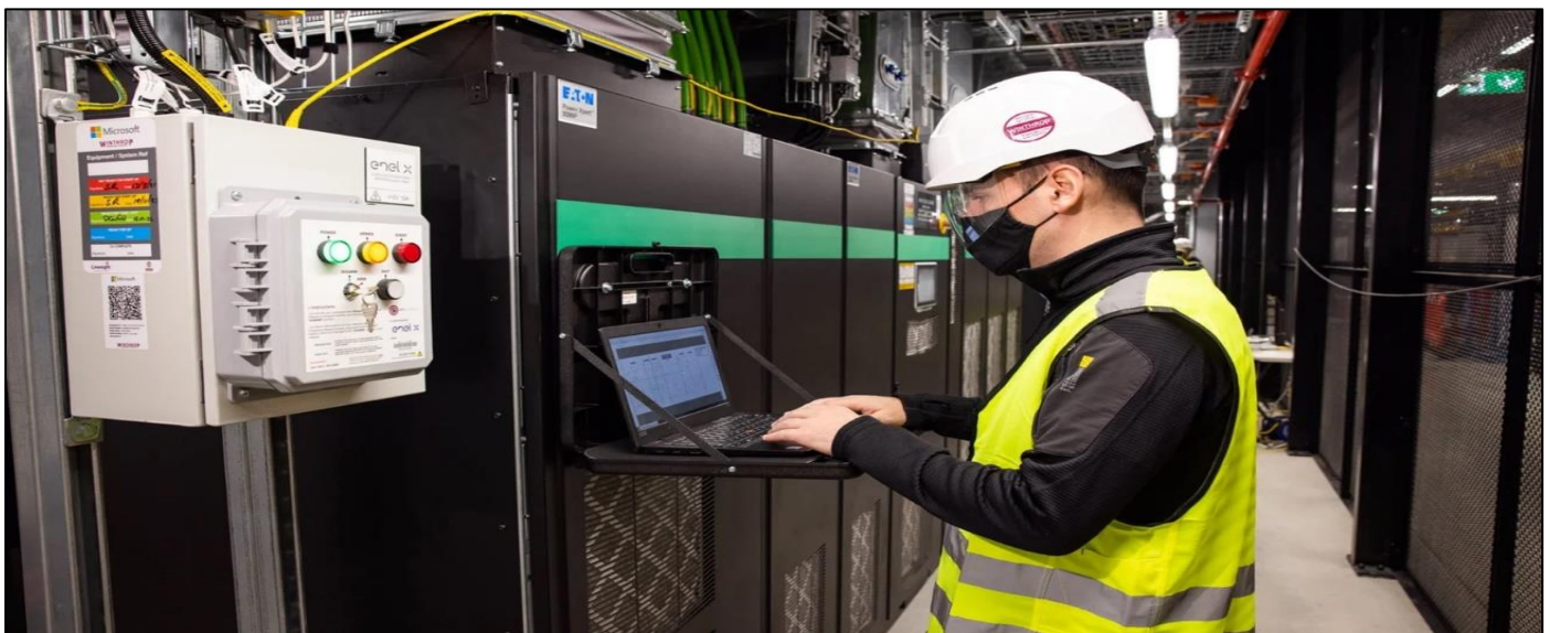
Fig 5 Maximizing Safety and Operational Simplicity in Radioactive Battery Management: Digital Monitoring with Full PPE Compliances
